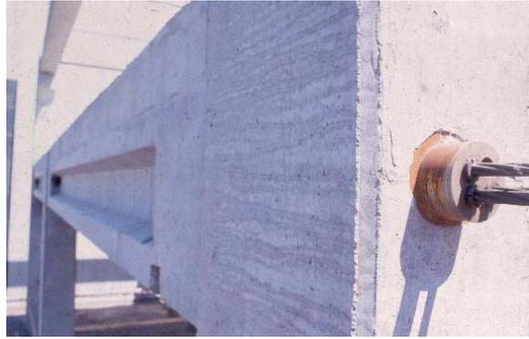
Figure-3: Full Scale Post-Tensioned Connection
