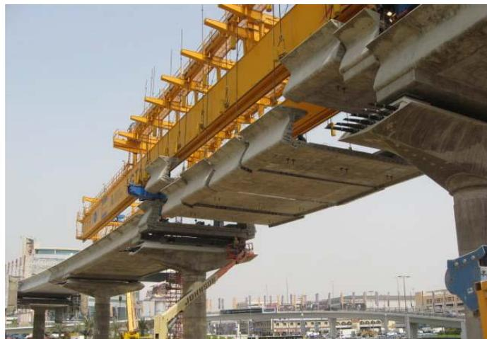
Picture 9: Launching gantry during segment geometry adjustment
