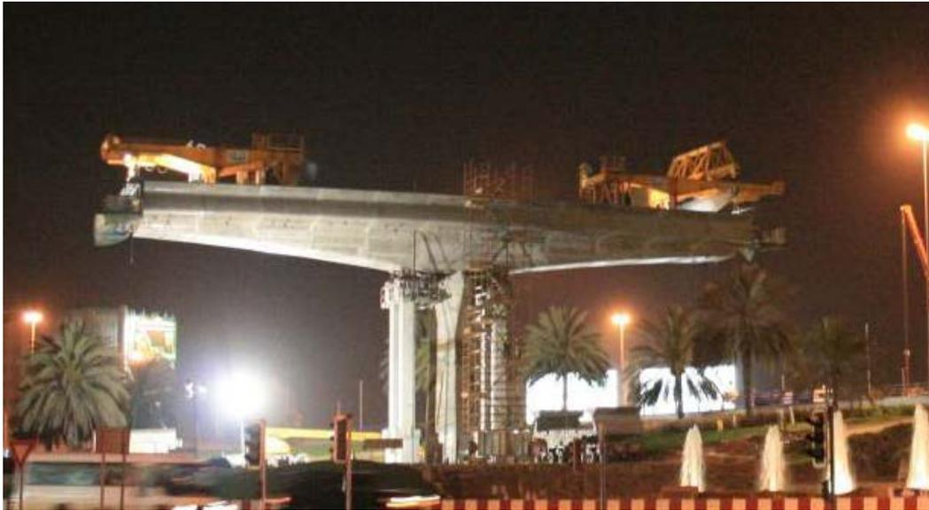
Picture 11: precast segment balanced cantilever erection method
