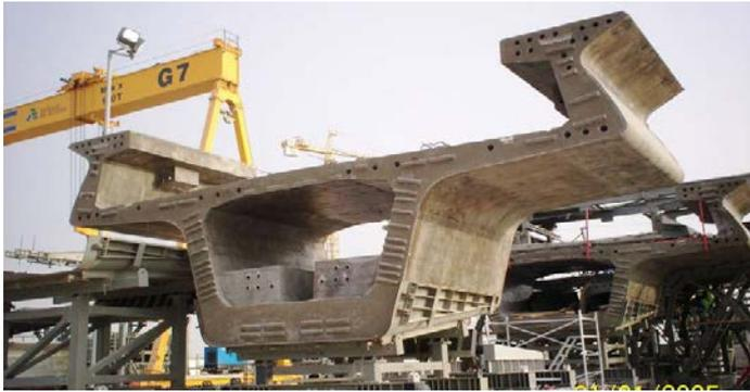
Picture 7: Typical balanced cantilever at casting area
